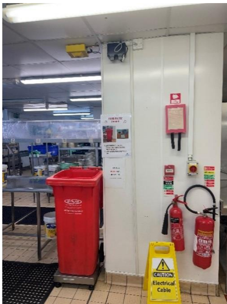
Figure 9 Positive Carbon bin in the Hudson Bay Hotel kitchen
